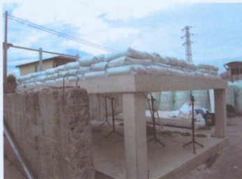
Photo of floor load arrangement (up to 250 kg/m 2 )
