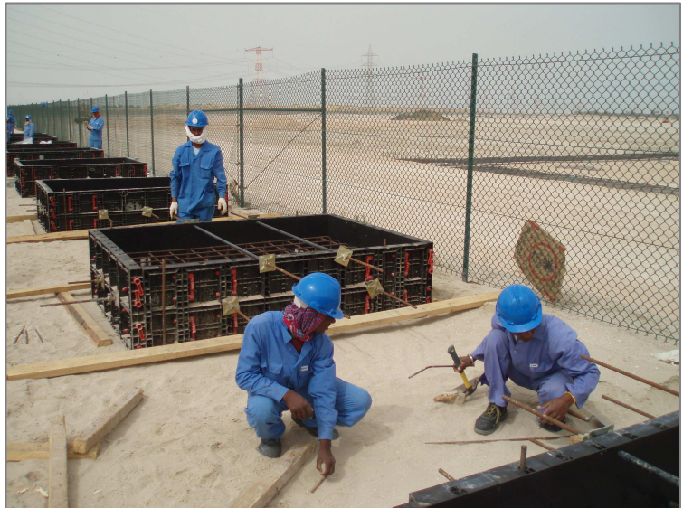
Example of pile cap with tie-rods and base-fixing
